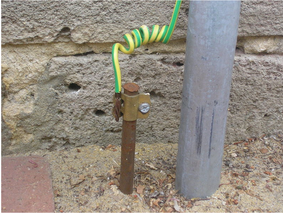
Typical Copper Earth of a Household
