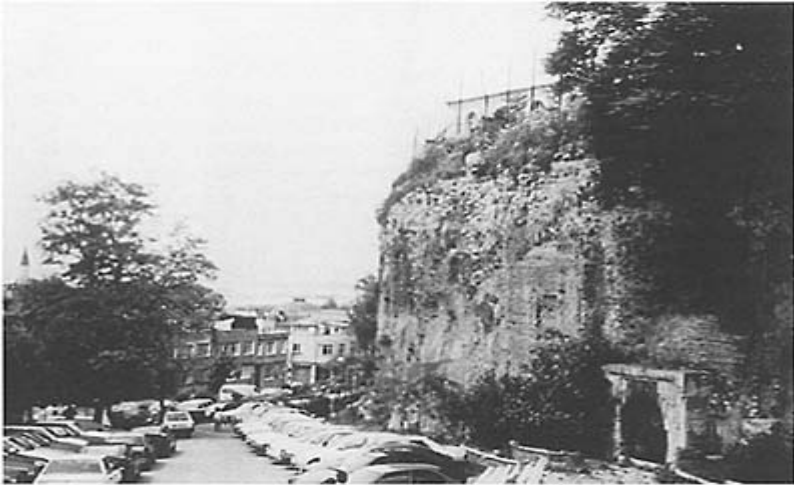
Ill. 74 The 20-meter-high stone buttressing for the seats at the south end of the hippodrome above the Sea of Marmora.
