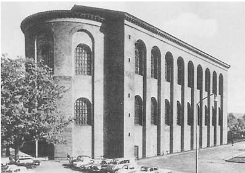
Ill. 19 Exterior of the northern apse and western side of the palace audience hall of Constantine at Trier.
