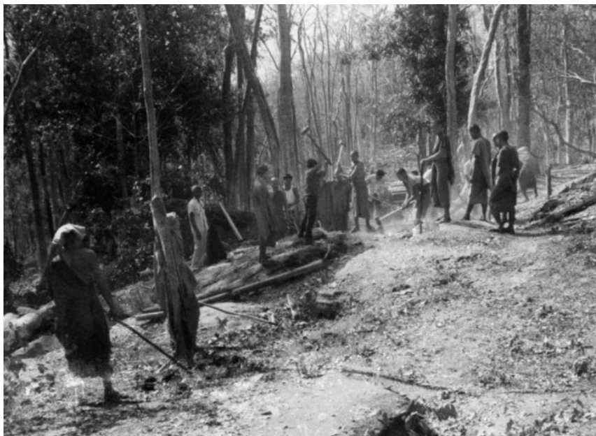
Construction of the road to Wat Tam Saeng Pet. See page 429.
